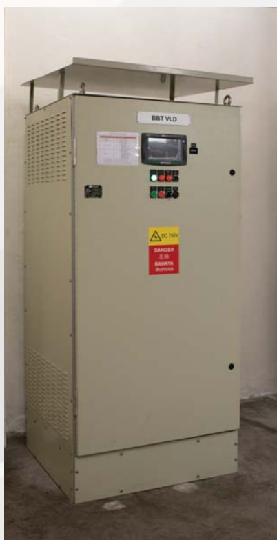
Voltage Limiting Device to isolate faults to a limited sector of a track.
